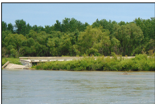
Highway 12 Bridge break after the 2019 Bomb Cyclone.
